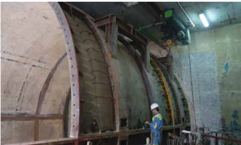
Above: Steel bell comprising heavy, but still manageable components
